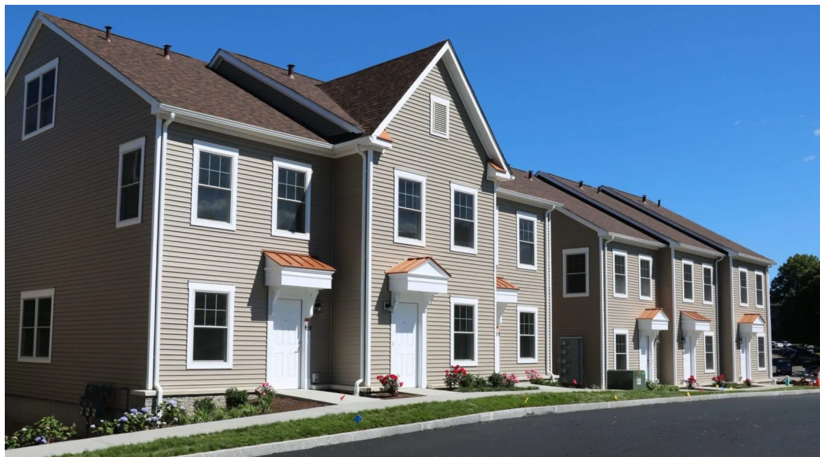
A few of the 18 new affordable housing units built by Greenwich at Armstrong Court.
