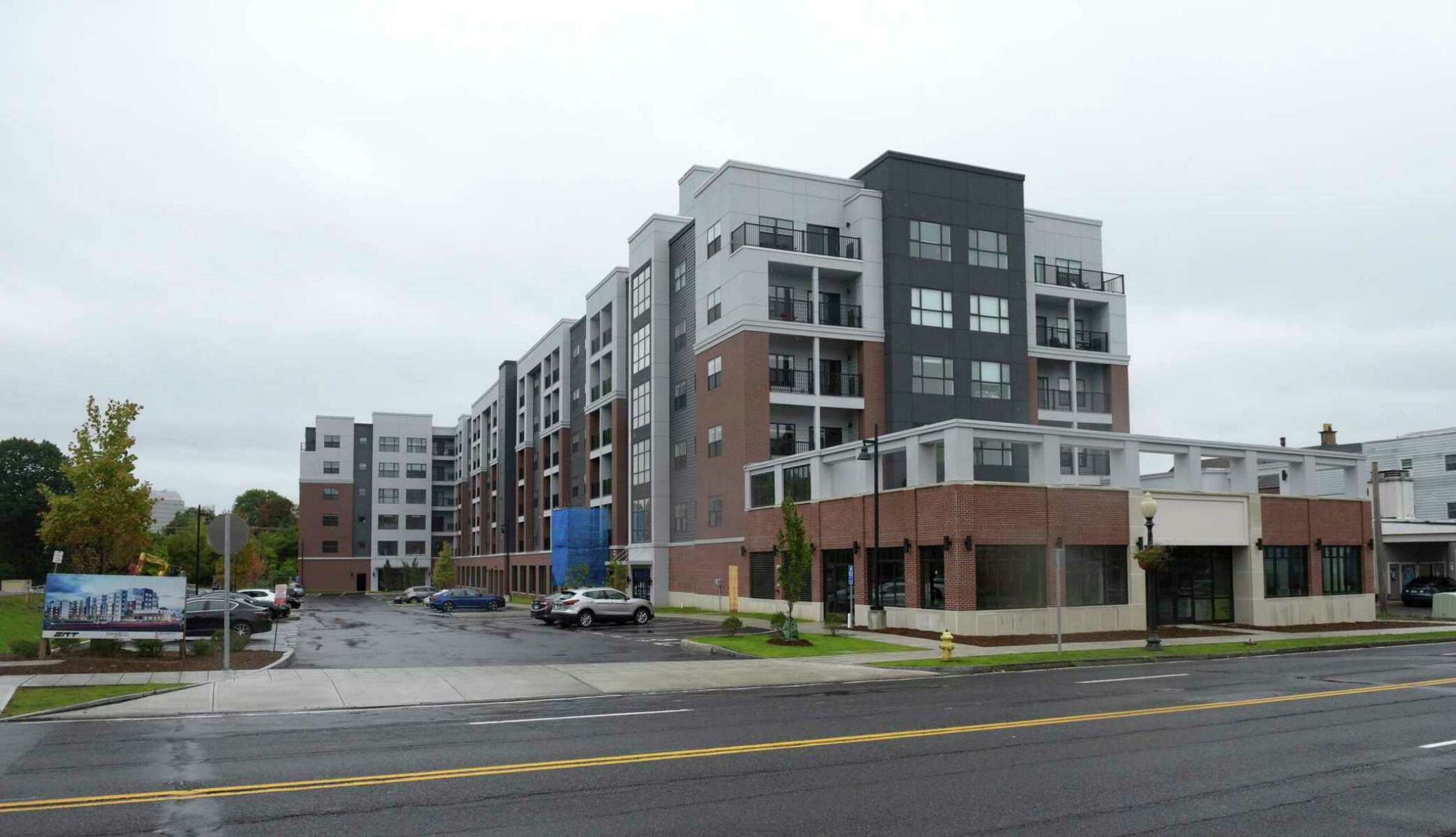
149-unit apartment building under construction at the former News-Times building at 333 Main Street, in Danbury, Conn. Tuesday, October 4, 2022.
